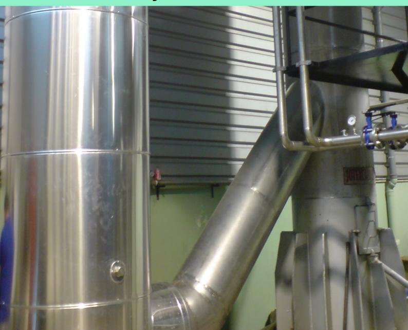
High performance heat recovery from flue gas of gas heated steam boilers
