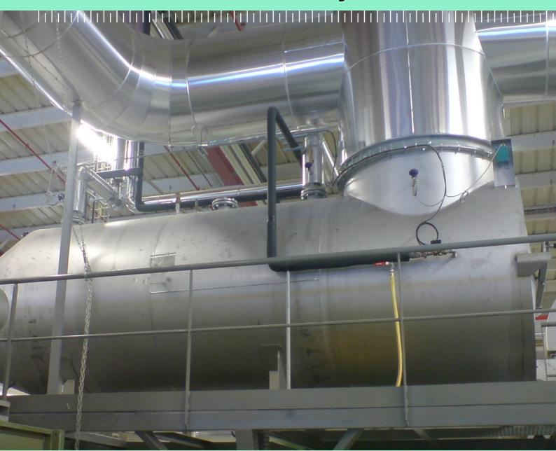
High performance air to water heat recovery system for exhaust air systems, stenter frames and driers
