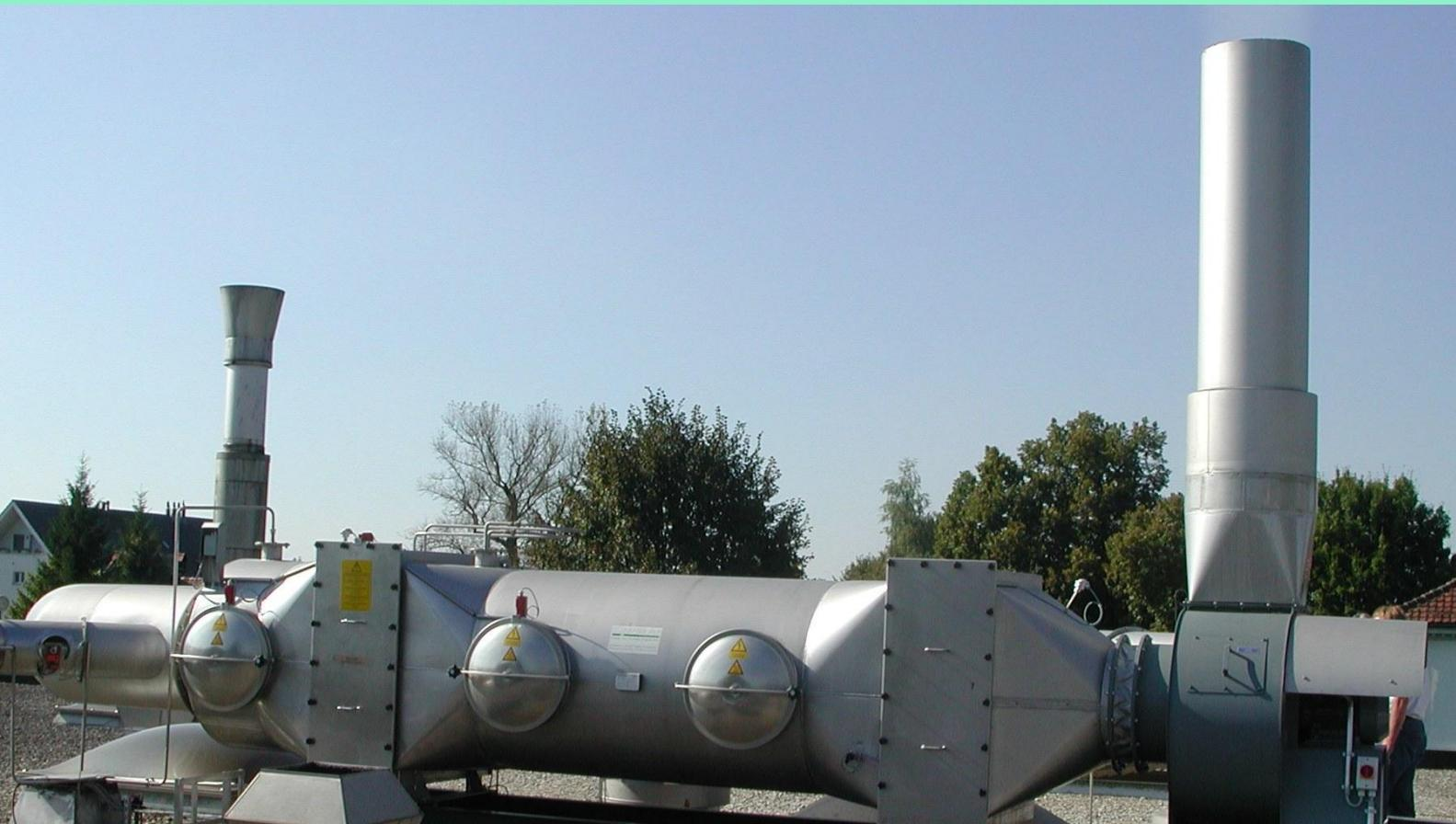
High performance Air Cleaning Systems for polluted exhaust air systems, stenters frames, coating machines and dryers
